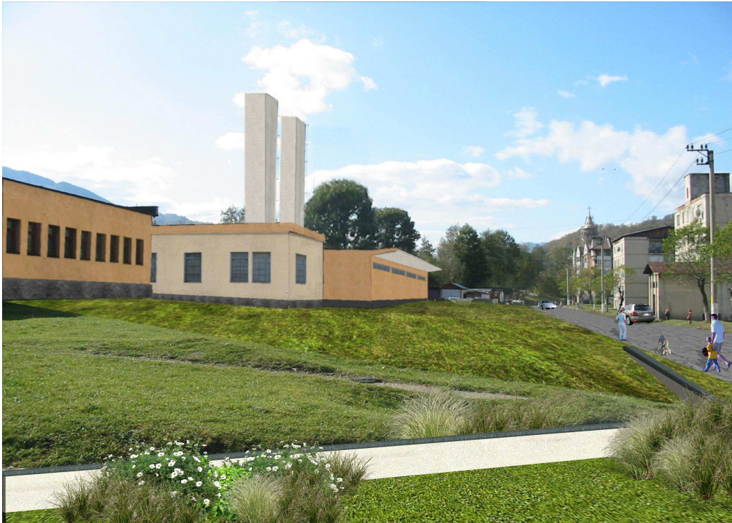
Fig. 2 - Bucura 1 Thermal plant after rehabilitation
