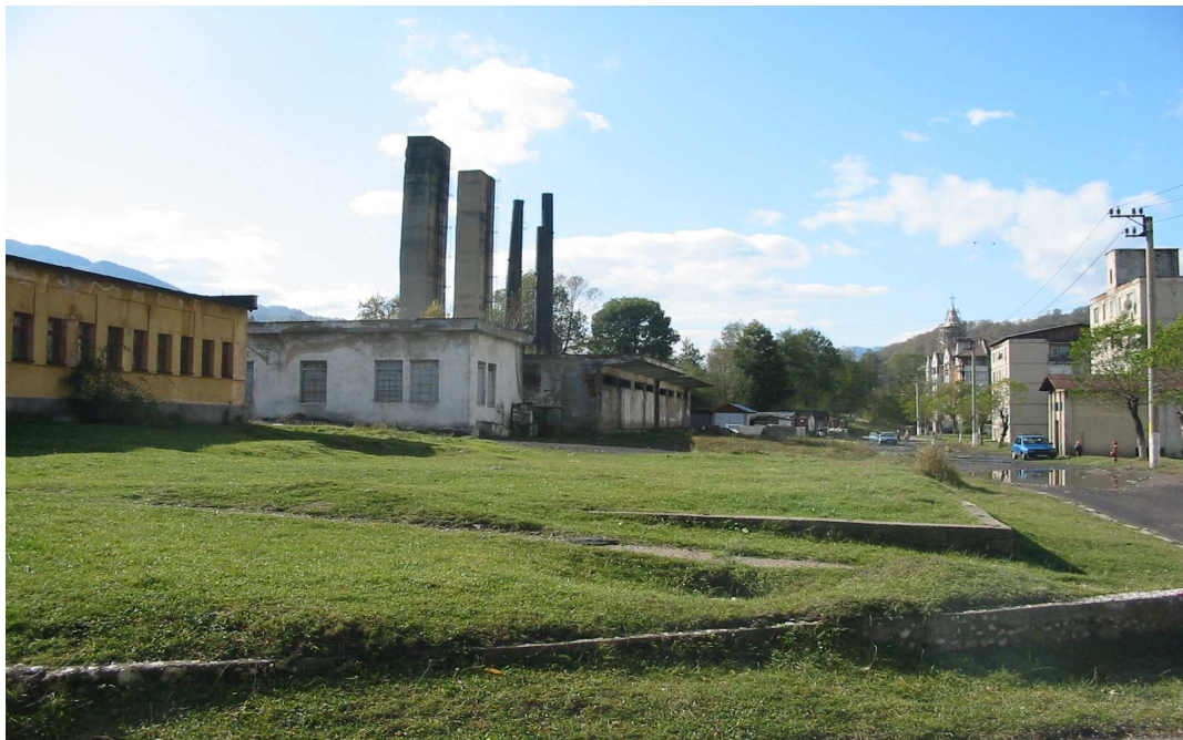
Fig. 1 - Bucura 1 Thermal plant 1 before being rehabilitated
