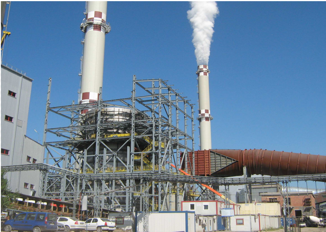
ROVINARI TPP. Desulphurisation plant. Absorber block 6 Rovinari
